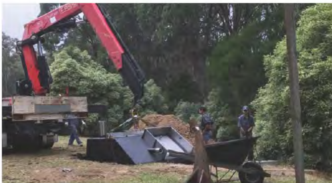
BUNKER BEING CRANED INTO POSITION RADY FOR INSTALL
