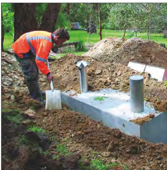
Compacting by hand.
