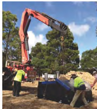
BUNKER BEING CRANED INTO POSITION RADY FOR INSTALL
